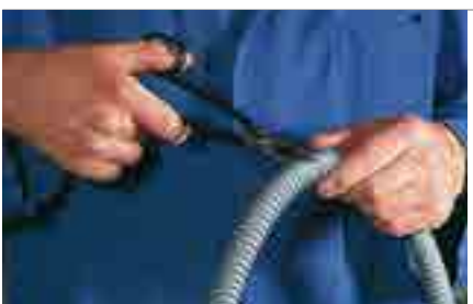
Kunststoff-Ummantelung durchschneiden Cut through the plastic sheathing
